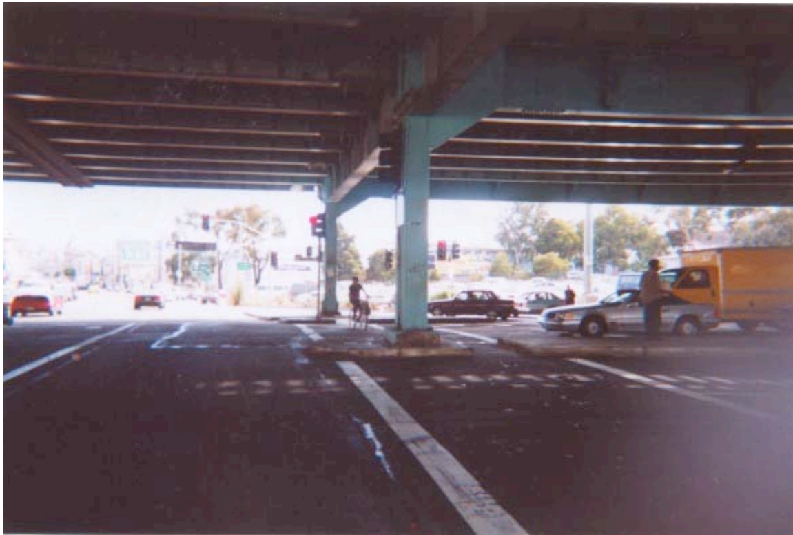
Figure G: passing under Route 101 superstructure
