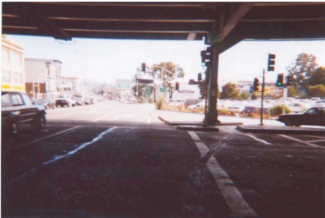
Figure H: entering into the double turn-lanes
